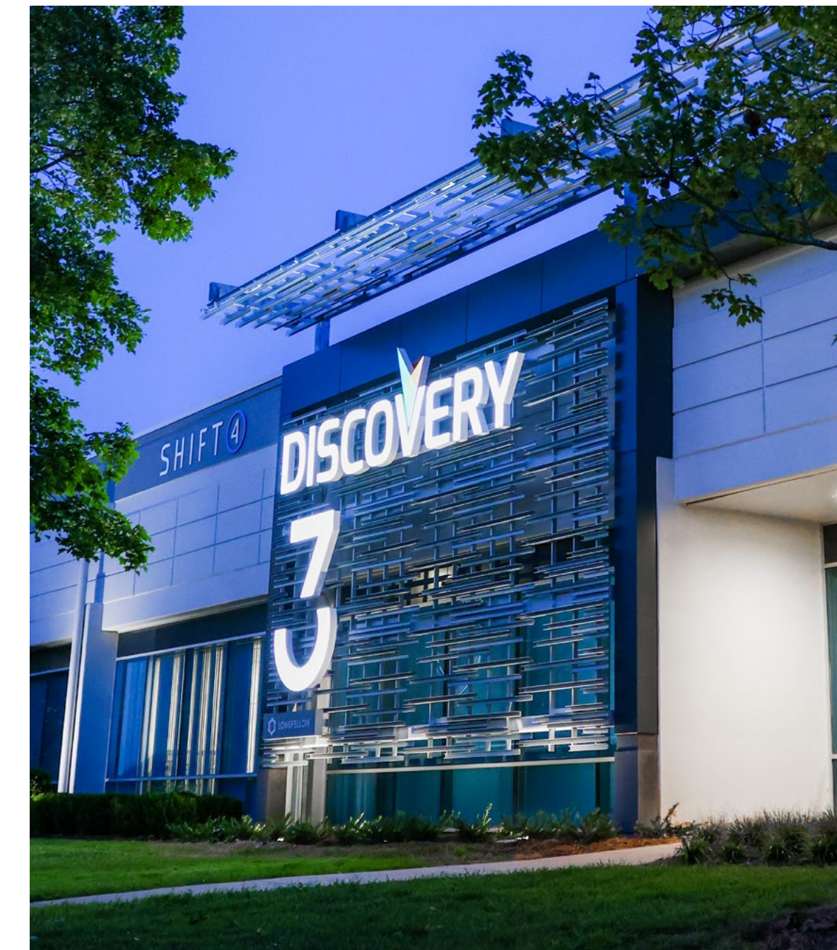
2 DISCOVERY AT PERIMETER MORRISVILLE, NC
